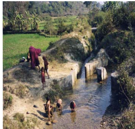
Figure 3: Main Canal of KUIS
