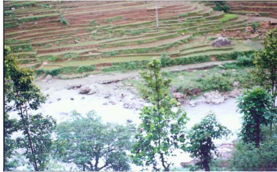
Figure 7: Side Intake Parewatar Irrigation System, at Thoppal Khola, Dhading District
