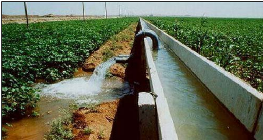
Figure 3: Typical Canalette and Siphon Used for Abstraction Water to the Field
