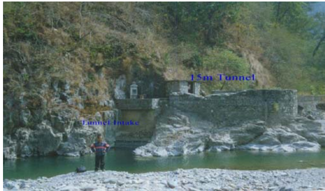
Figure 8: Tunnel Side Intake of Rampurphant Irrigation Project at Nisti Khola, Palpa District
