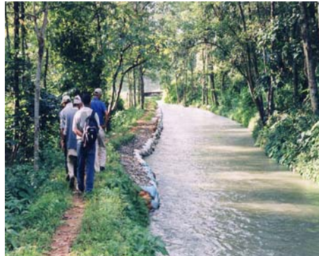
Figure 4: Main Canal of BIP
