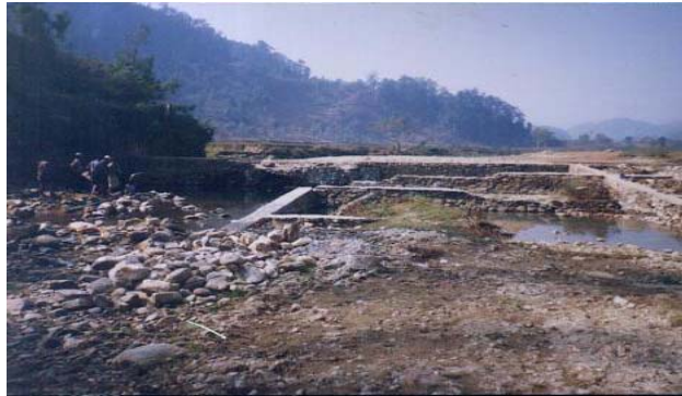
Figure 3: Sange Patyani Irrigation System, Tanahu
